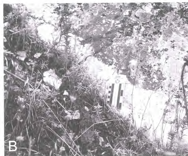
Fig. 11 – a) free-face due to primary surface faulting along the bedrock fault scarp near Costa Monticello; b) detail of the 1980 coseismic reactivation (vertical offset nearly 20 cm). Location is slightly west of the site of Fig. 10. Mr. Ferracane (left) witnessed the event and provided precious information.
