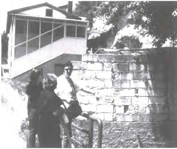
Fig. 7 - Costa Pannicaro site (B in Fig. 2; arrows in Fig. 6), Sabina points to a broken wall which suffered a vertical displacement of nearly 20 cm, being located right above the 1980 fault rupture; the old woman witnessed the event.
